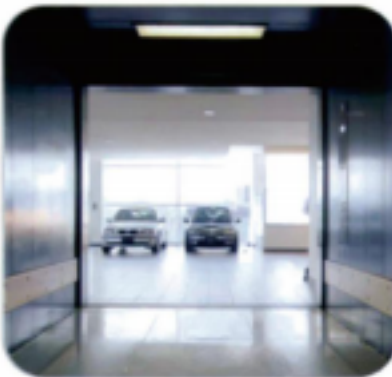
⌘ Front-and-rear opening elevator car
